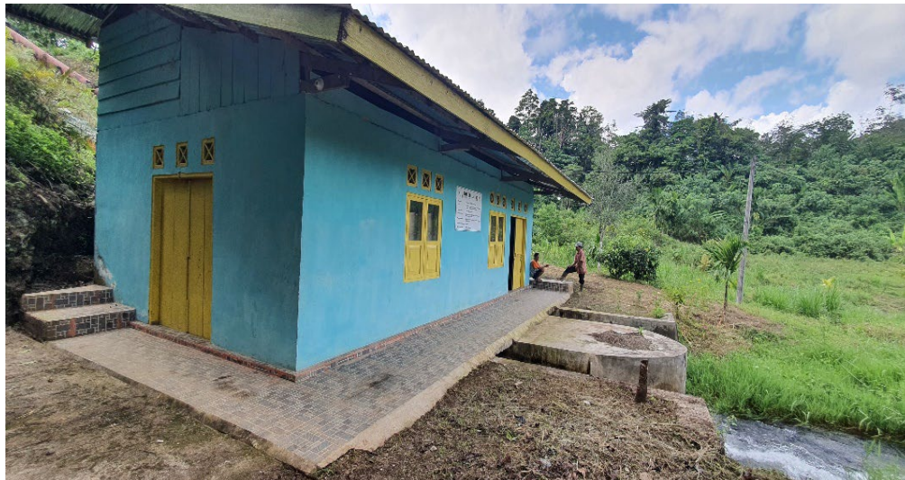
Figure 14: Interior and Exterior of MHP Turbine House
