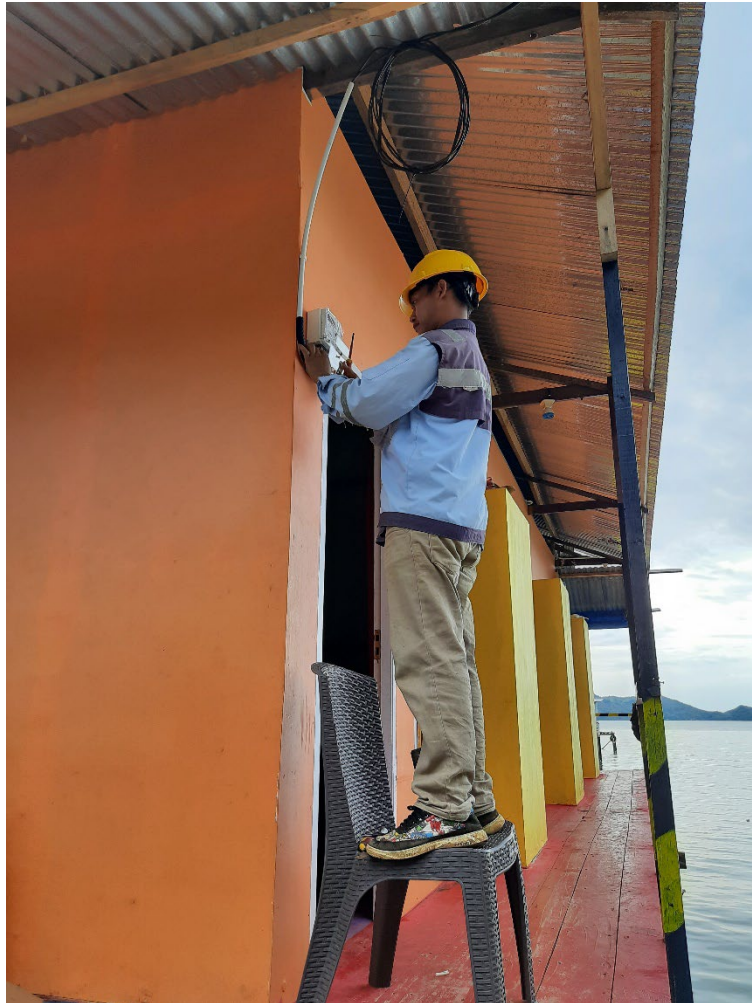
Figure 13: SPV Technician Installing a New Connection
