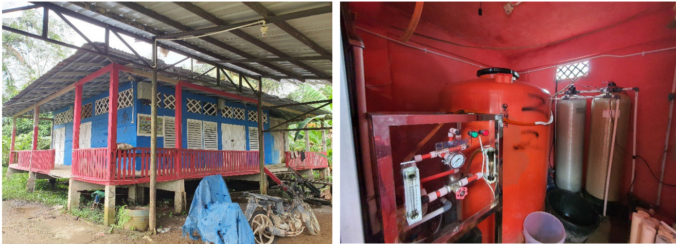
Figure 20: Water Purification Production House in Sungai Rambut
